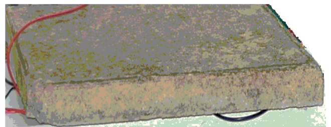
Figure 1.a First Image of slab using mobile camera
